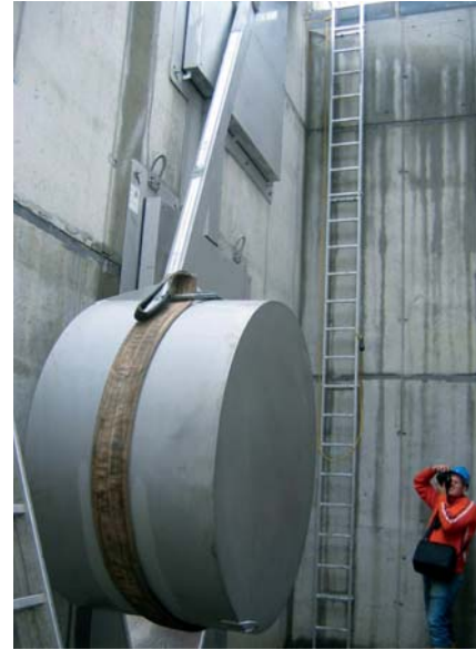
Fig. 5: HydroSlide® flow regulator
