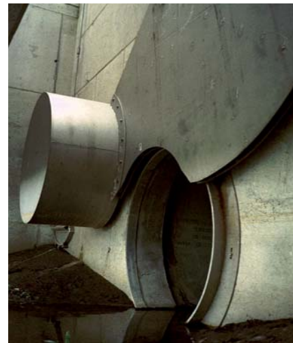
Fig. 7 HydroSlide® flow regulator
