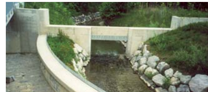
Fig. 6: HydroStyx® flow brake
