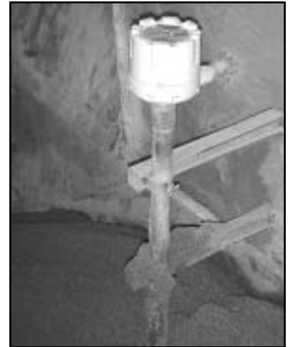
An installed SafePoint ® unit in an aggregate application.
